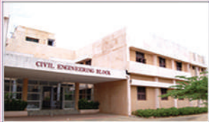
Civil Engineering Block
